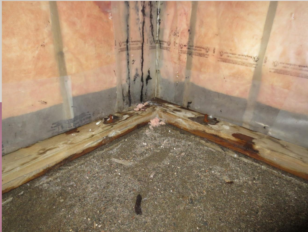
Walls damaged by moisture & mold. Picture courtesy of Michael McKay
