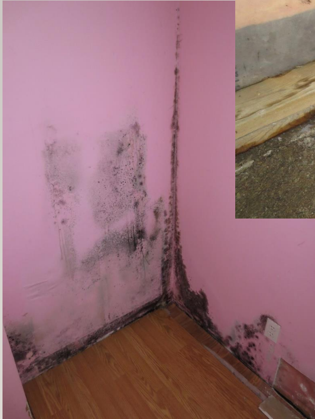
Walls damaged by moisture & mold. Picture courtesy of Michael McKay
