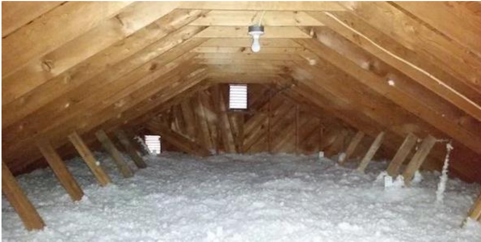
Ceiling with Attic Space
